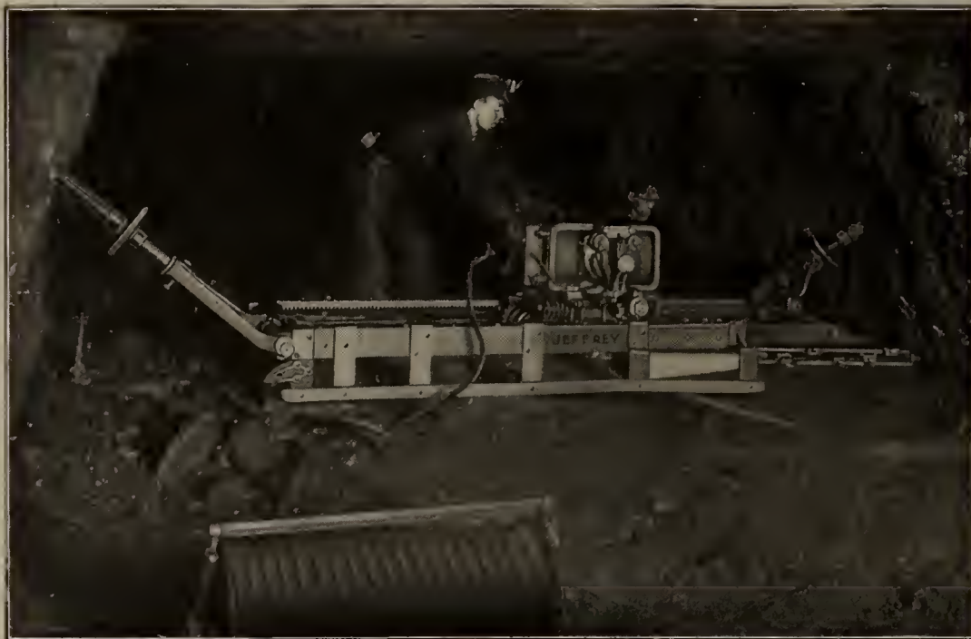
17A ELECTRIC CHAIN COAL CUTTER AT WORK.
